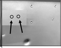
52) Attach door closure to bracket on door with pin (provided with closure). NOTE: adjust closure speed by turning cylinder (Instructions for turning direction are on cylinder "small print"). A minimum of 5 seconds required for door to close.
