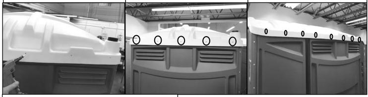
40) Rivet roof to front door frame. Pull roof down & transfer drill through holes in roof into top door frame facing use #10 (.193") [5 mm] Drill bit. (DO NOT to drill through 2<sup>nd</sup> wall of facing) Rivet roof to front top facing with (6) rivets PN 22604.
