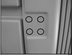
50) Rivet door closure bracket to door (included with door closure). Install bracket completely to the left using (2) rivets PN 17436 Add 3<sup>rd</sup> rivet far left of bracket, drill hole through bracket into door using #10 (.193") [5 mm] Drill bit.
