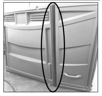
11) Install (1) rivet P/N 22604 from inside unit through bottom panel hole into bottom stiffener tube hole. Install remaining (7) rivets PN 22604. *Note: Hold Rivet-gun square to surface being riveted. Press stiffener tube firmly against panels.* Repeat steps 10 & 11 on Right half panel to Right side panel. Position the Right half panel to Right side panel *(right half panel overlaps right side panel).*
