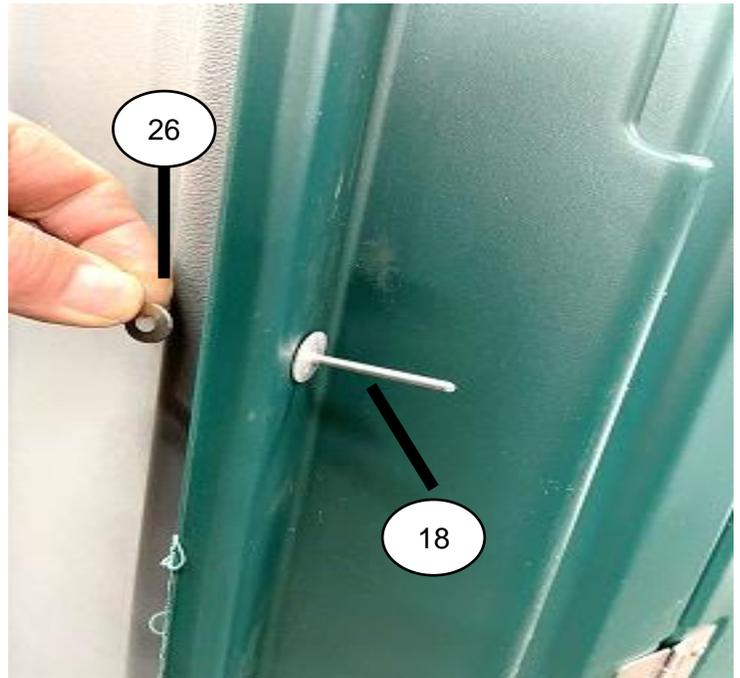
Tip unit up on base & place front against side panels with edge of panel tucked in groove on inside edge of front. Align holes in front with holes in panels & use 1 rivet #11054 on front & 1 washer #11315 on panel in middle in holes on left & right side of front.
