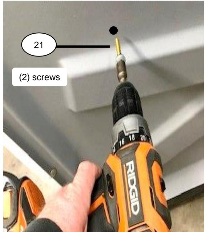
Locate 2 dimples in lower section of rear panel. Install (2) Screws #13860 through dimples into tank using of 3/8" Nut Driver bit.
