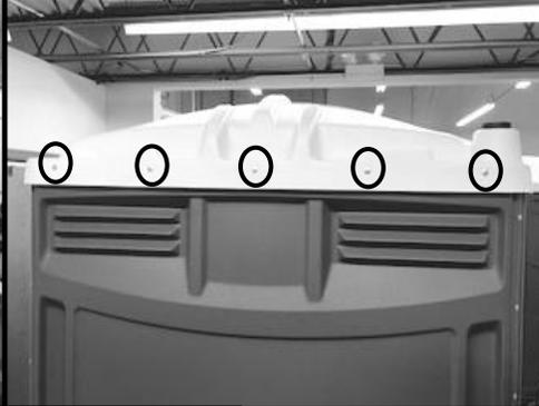
39) Rivet roof to side panels using (8) rivets P/N 11054 per side installed from outside of roof and (8) washers P/N 11315 per side inside unit on rivets.
