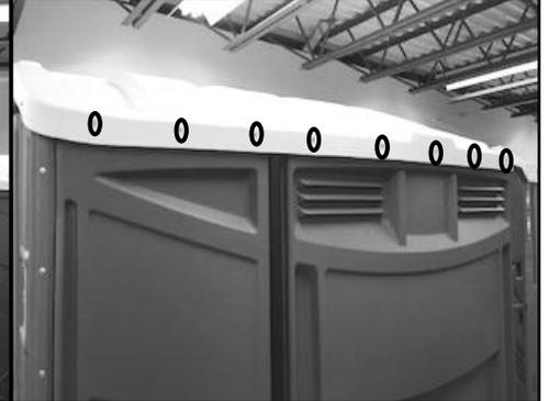
40) Rivet roof to front door frame. Pull roof down & transfer drill through holes in roof into top door frame facing use #10 (.193") [5 mm] Drill bit. **(DO NOT to drill through 2<sup>nd</sup> wall of facing)** Rivet roof to front top facing with (6) rivets PN 22604.
