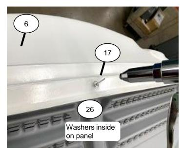
At rear of roof start at center hole location. Fasten roof to rear panel using Rivet #11030 outside on roof & Washer #11315 inside on panel.
